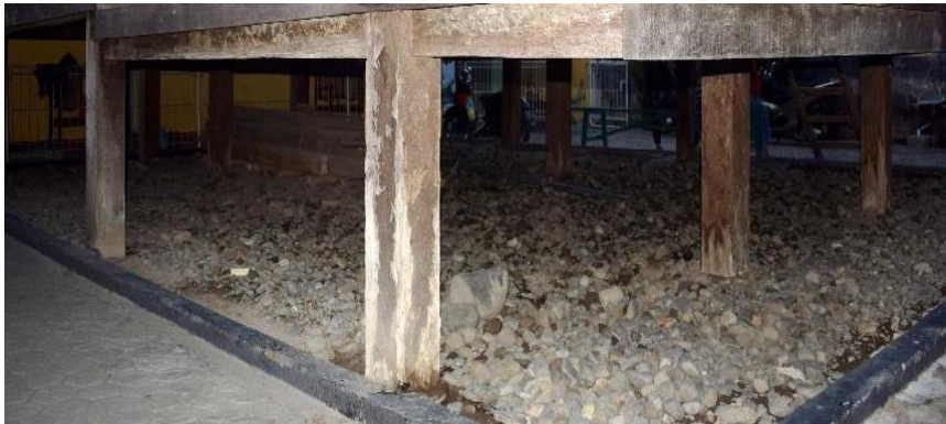
Figure 3. The Pillars of the Panjalin Traditional House
