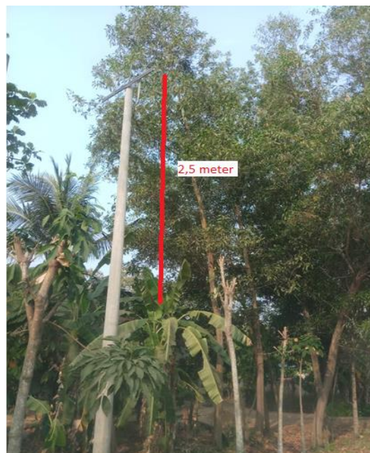
Figure 4. The distance between poles and trees.
